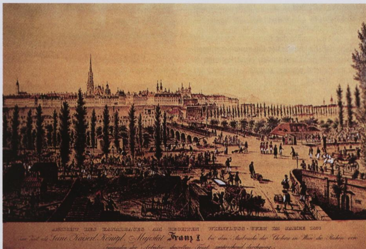
Fig. 3, Start of construction works for Right Wien River Collector, autumn 1831
