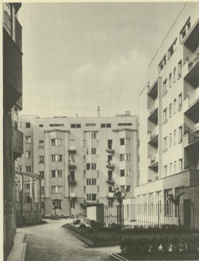
„Südtirolerhof“ (South Tyrol Buildings), IV., Wiednergürtel 38/40 (185 flats) Tram: Ring—Oper/66, 67/18G, 118 Design: Hahn & Ernst
