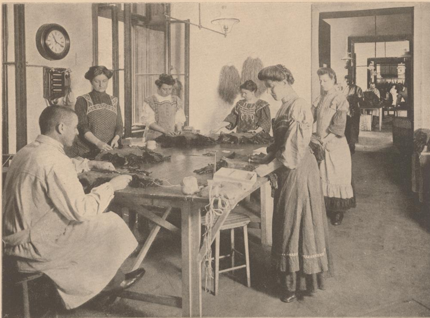
TYING THE PERSIANLAMB BUNDLES AND VIEW OF DIFFERENT SORTING ROOMS.
